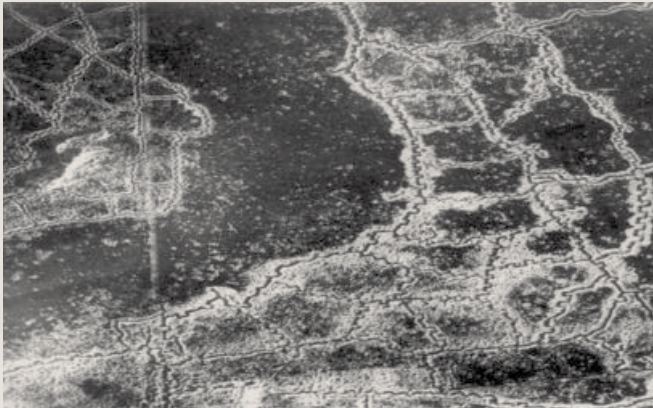
An aerial view of the extensive trench system
